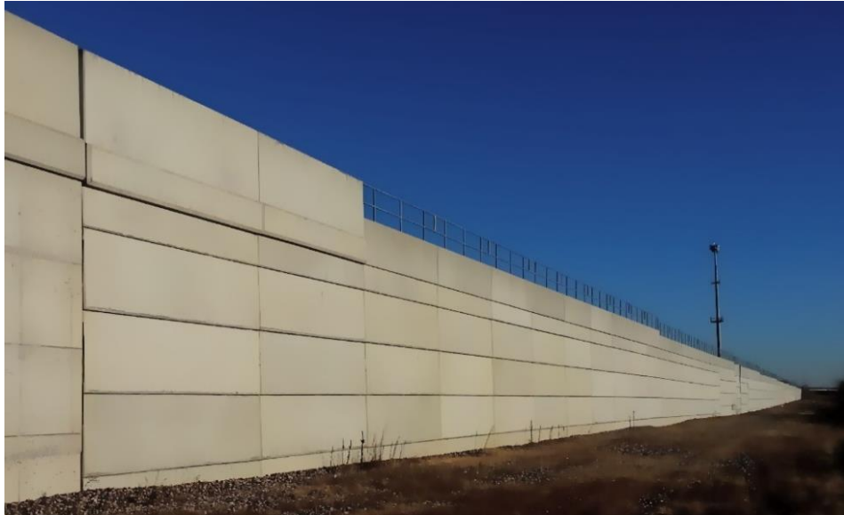
Gravity frame MAXI WALL built for BNSF in Olathe Kansas, the flagship of MAXI MSE Walls - 2000 elements
