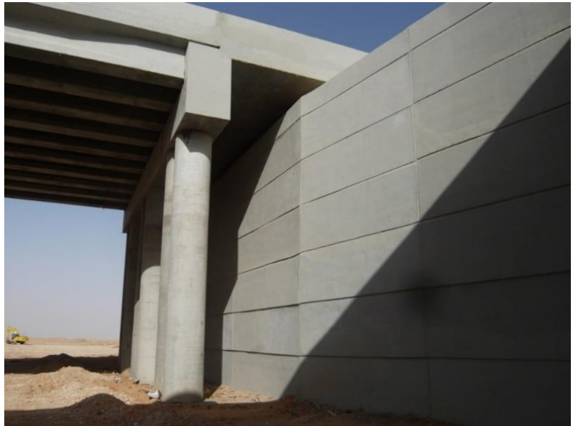
Vast experiences: 58 bridge abutments built for bridges across rails 373 miles, 600km long in Saudi Arabia.
