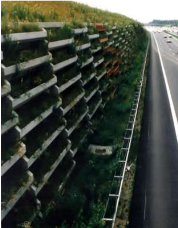
Raststatt GEO Wall after Construction
