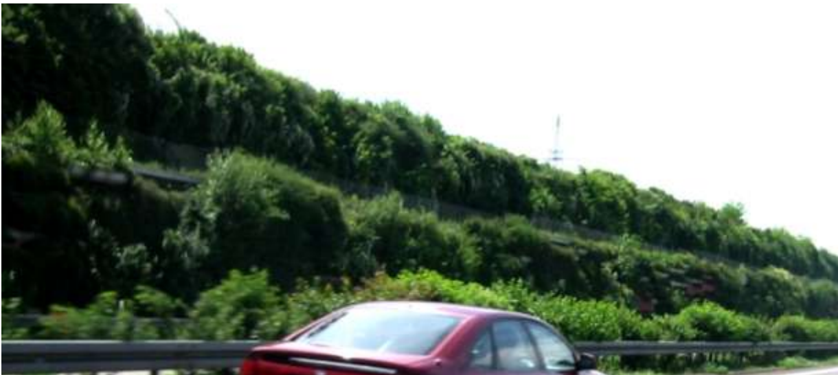
Evergreen GEO Retaining Wall (2 miles long) near Raststatt, Mannheim, Germany
