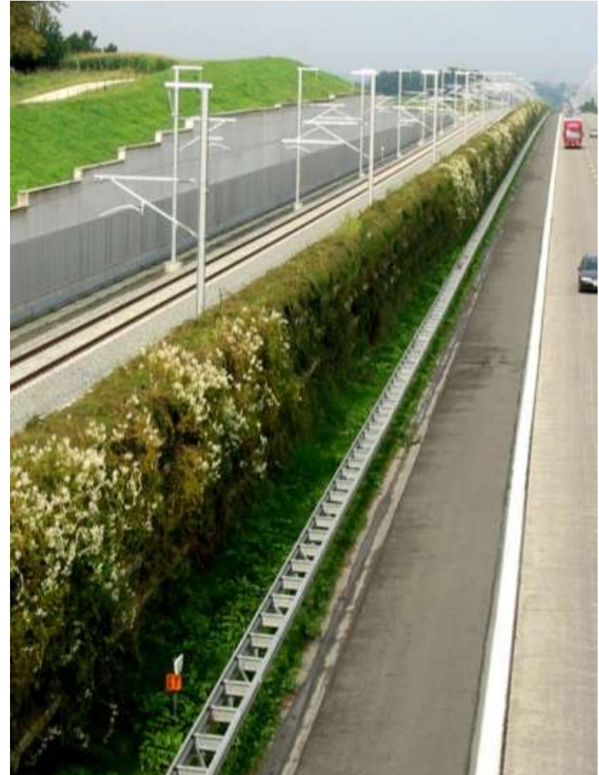
After one year; the longest wall ever built: 9 Miles.
