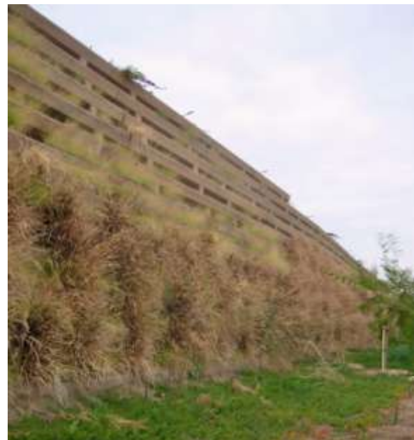
Spring Street San Diego I-92, for Caltrans
