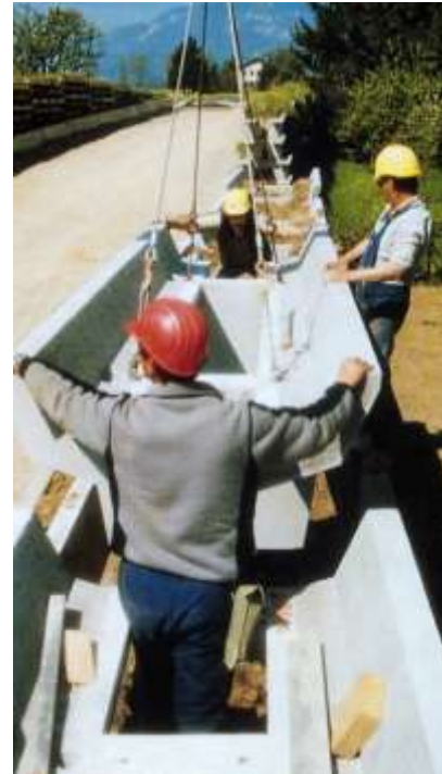
An excavator and three men set a unit in 3 minutes.
