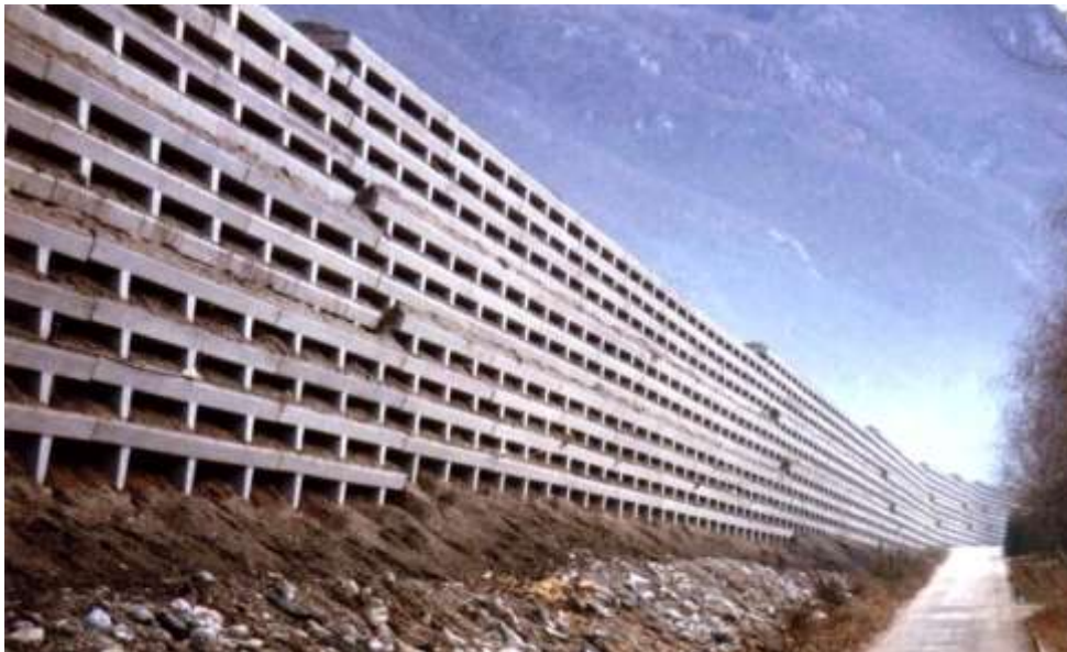
Sound Wall along Highway A2: After Construction and
