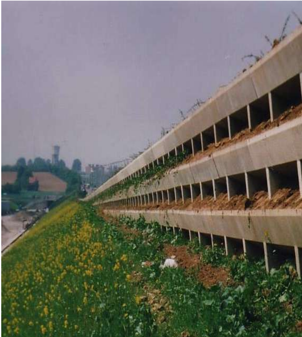
Bullet Train TGV Brussels - to Köln – Berlin under Construction:
