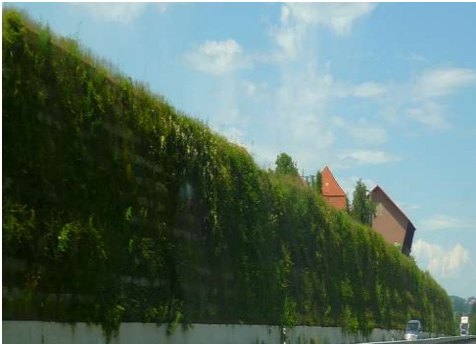
Evergreen sound wall along the Motorway A-2 in Switzerland
