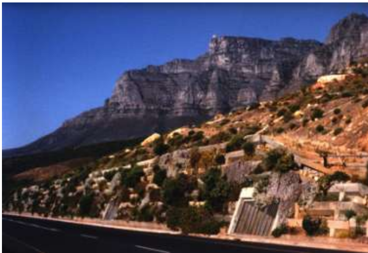
Evergreen Retaining wall stops a Landslide South Africa -
