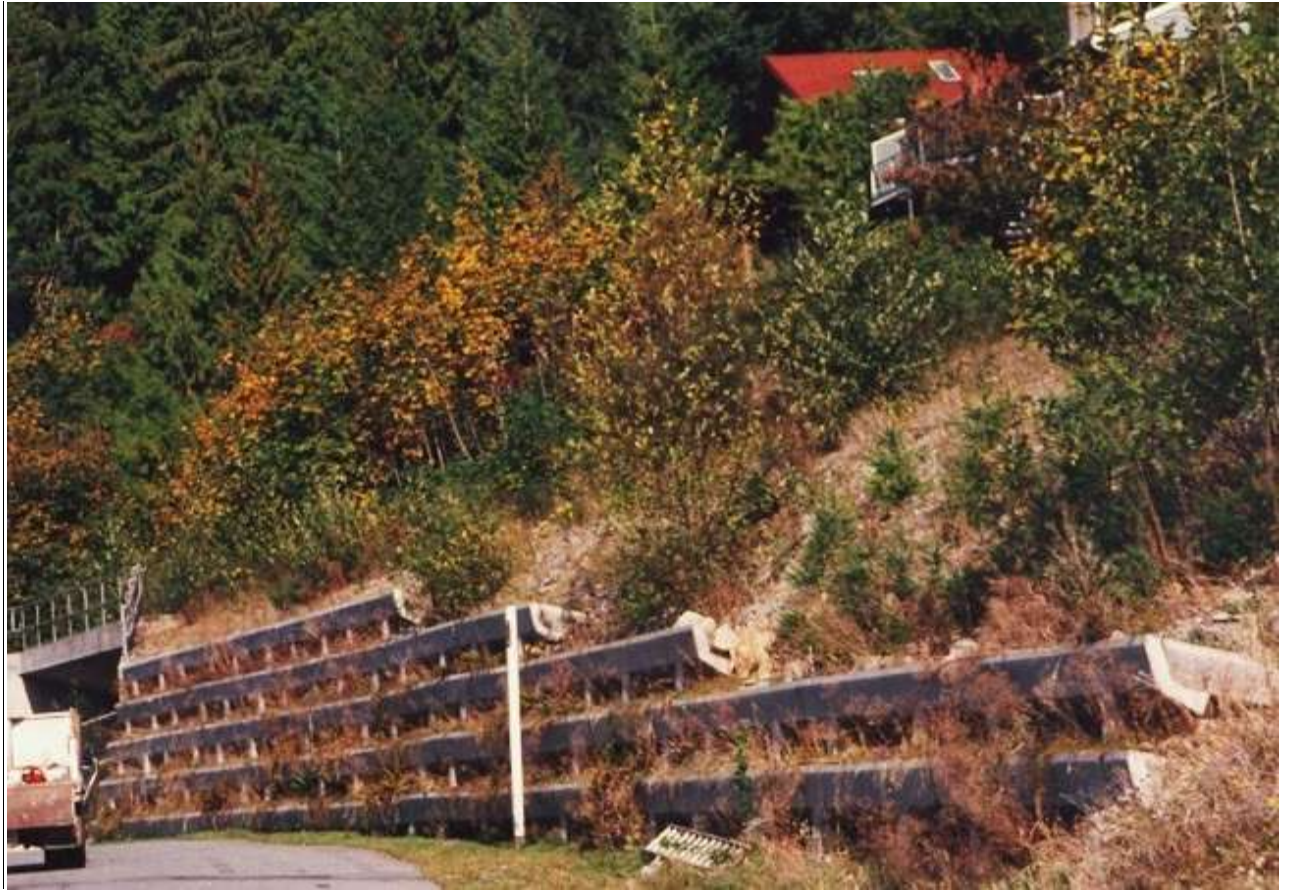
Evergreen Retaining Wall directly under British Columbia Rail Track
