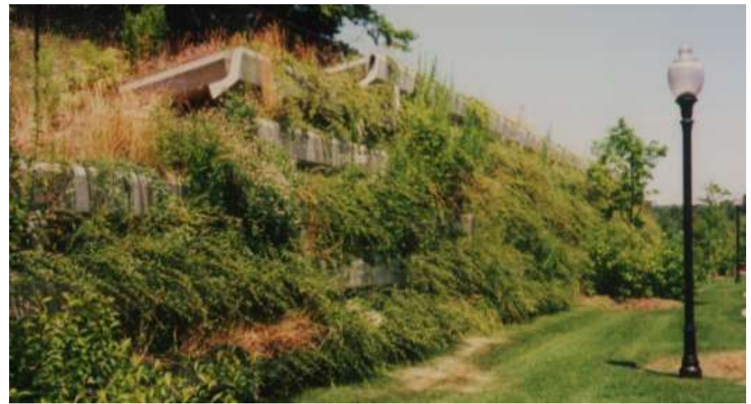
Retaining Wall in Smithtown, Long Island, NY
