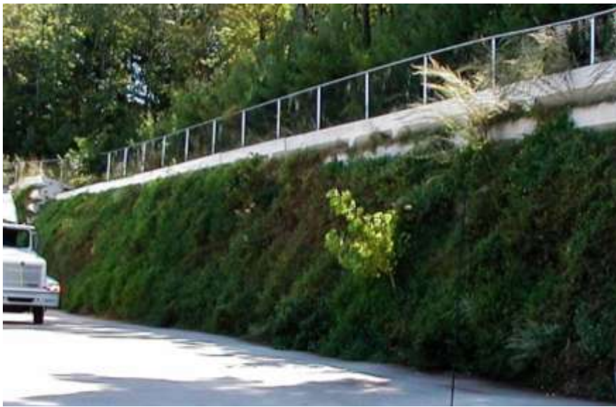
Natwick Shopping Center Retaining Wall, Boston
